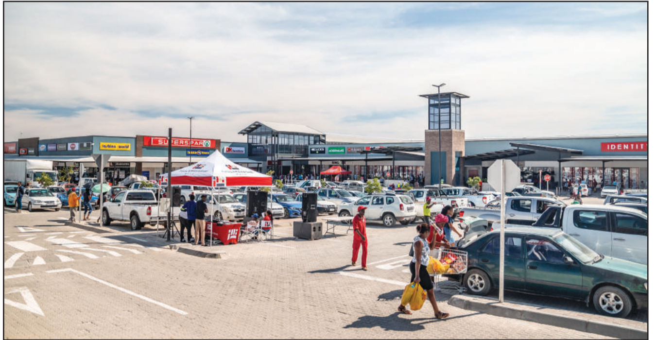
The newly built Thulamahashe Mall
